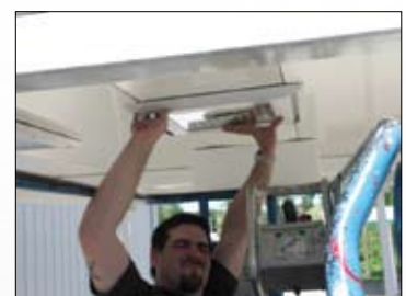
3. Insert Crossover fixture into the existing 4" hole & adapter panel.
