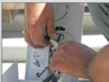
7. Make quick connect wiring connection inside box.
