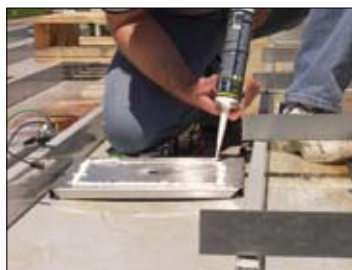
2. Apply specification-grade Crossover sealant to retrofit adapter panel (sealant and panel provided).
