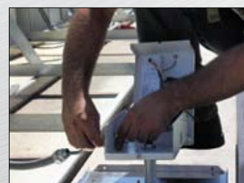
8. Attach existing conduit to driver box. Make necessary supply wiring connections inside the box. Close box.
