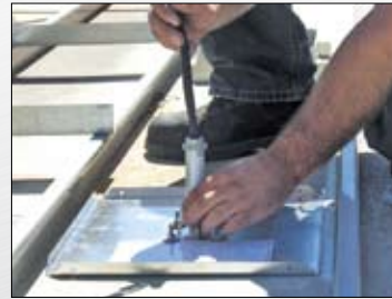
5. Feed quick connect wiring through 1-piece stem with attached washer, then screw stem onto fixture.
