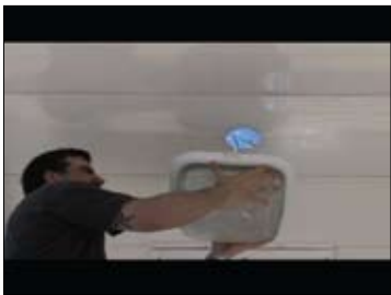
1. Remove existing Scottsdale fixture.
