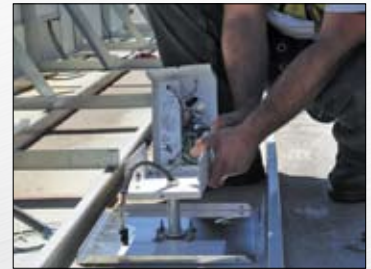
6. Open driver box and feed quick connect wiring through box. Secure box to 1-piece stem with lock nuts.
